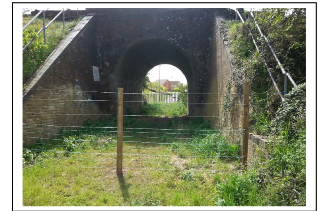
Photo 2: Alternative railway crossing - underpass
