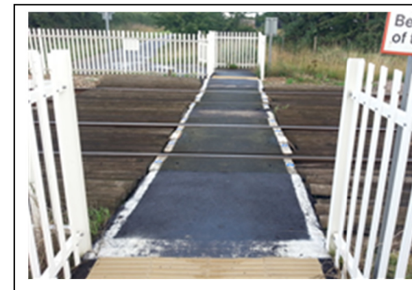
Photo 1: Existing level crossing - Cattishall
